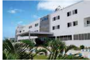
Rudrapur Plant (Green Building)
