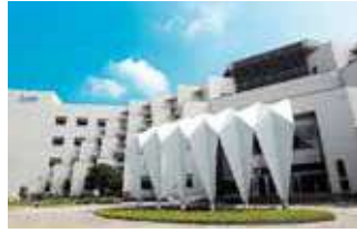
Tainan Plant (Diamond-rated Green Building)
